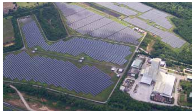
➤ Solar farm at Kaeng Khoi factory
